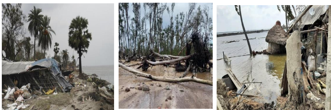
Fig. 1. Damage caused by Cyclone Amphan in May 2020 in Sundarban area of South 24 Parganas, West Bengal
