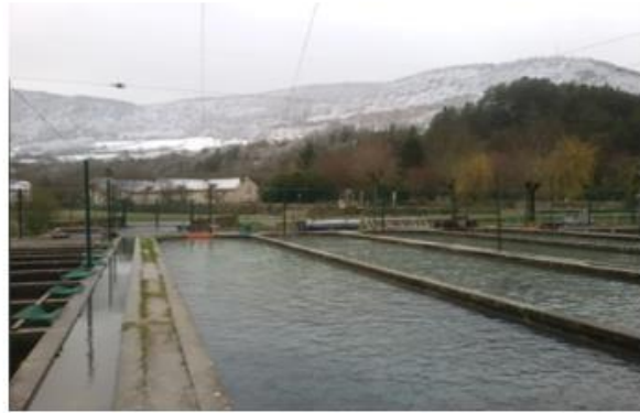
Fig. 1. Running water system constructed in a hilly region for cold water fisheries
